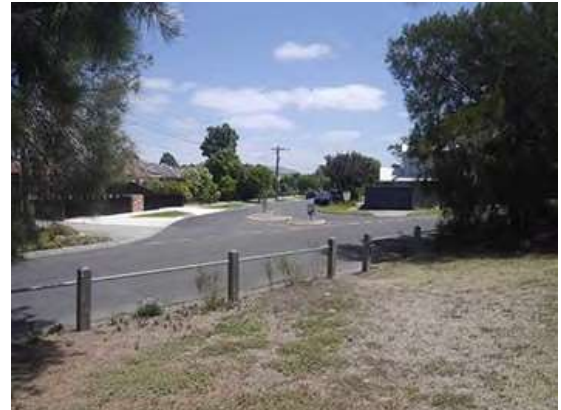
Photo 72: Bollard and rail fencing
