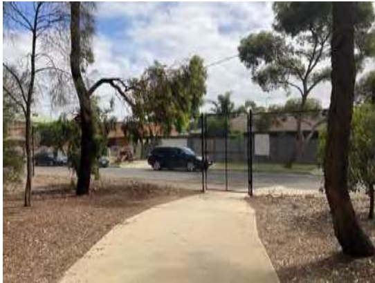
Photo 71: Chain mesh fence and gate
