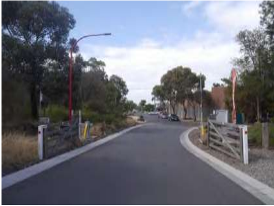
Photo 75: Timber vehicle entry gate
