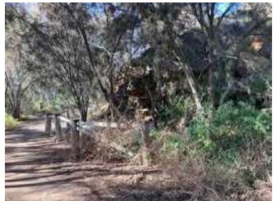
Photo 74: Timber post and rail fencing
