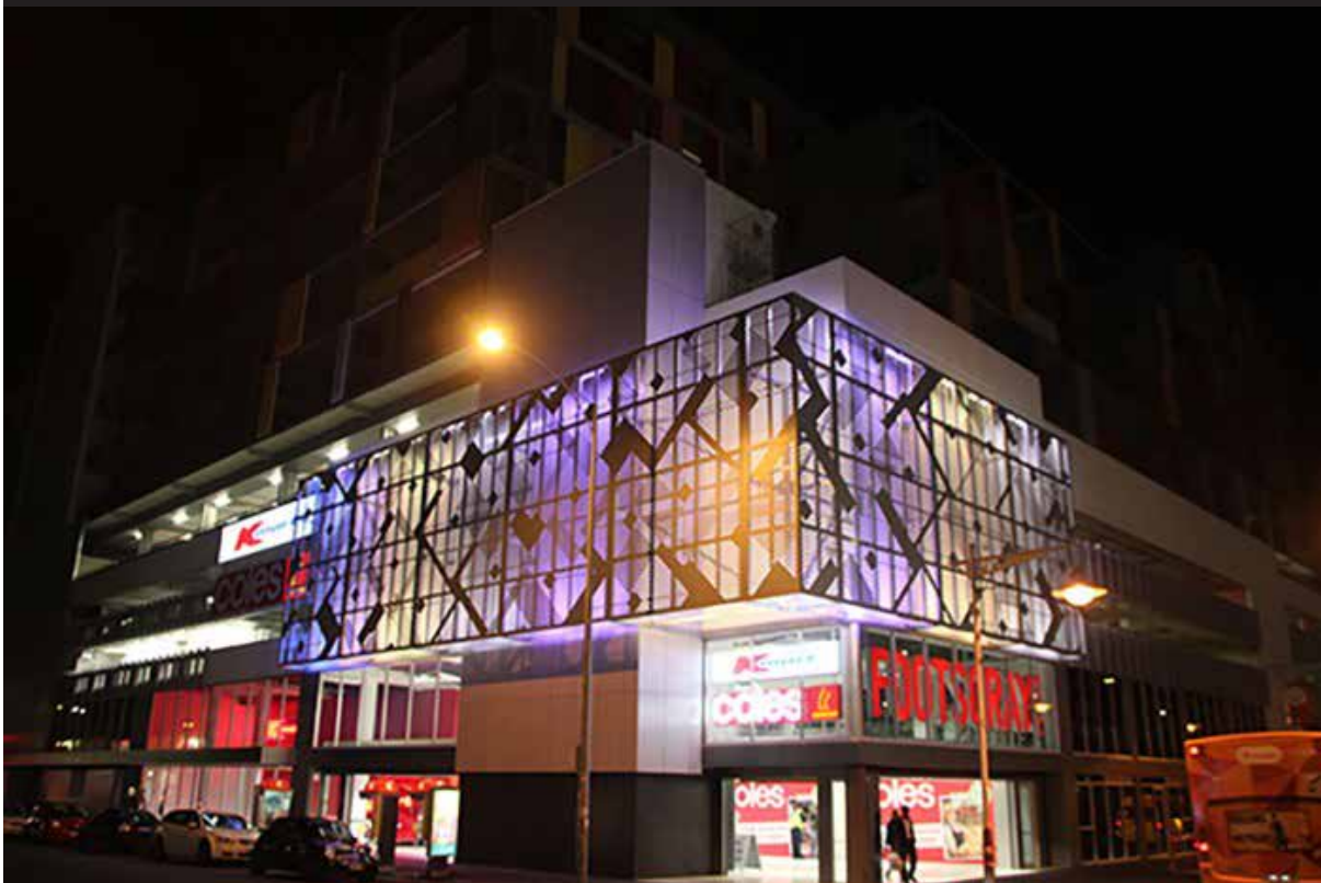
Footscray Plaza Artwork Facade, Matthew Harding Footscray, VIC 2014 Aluminium and LEDs. Approx. 250 square meter http://matthewharding.com.au/work/footscray-plaza-artwork-facade
